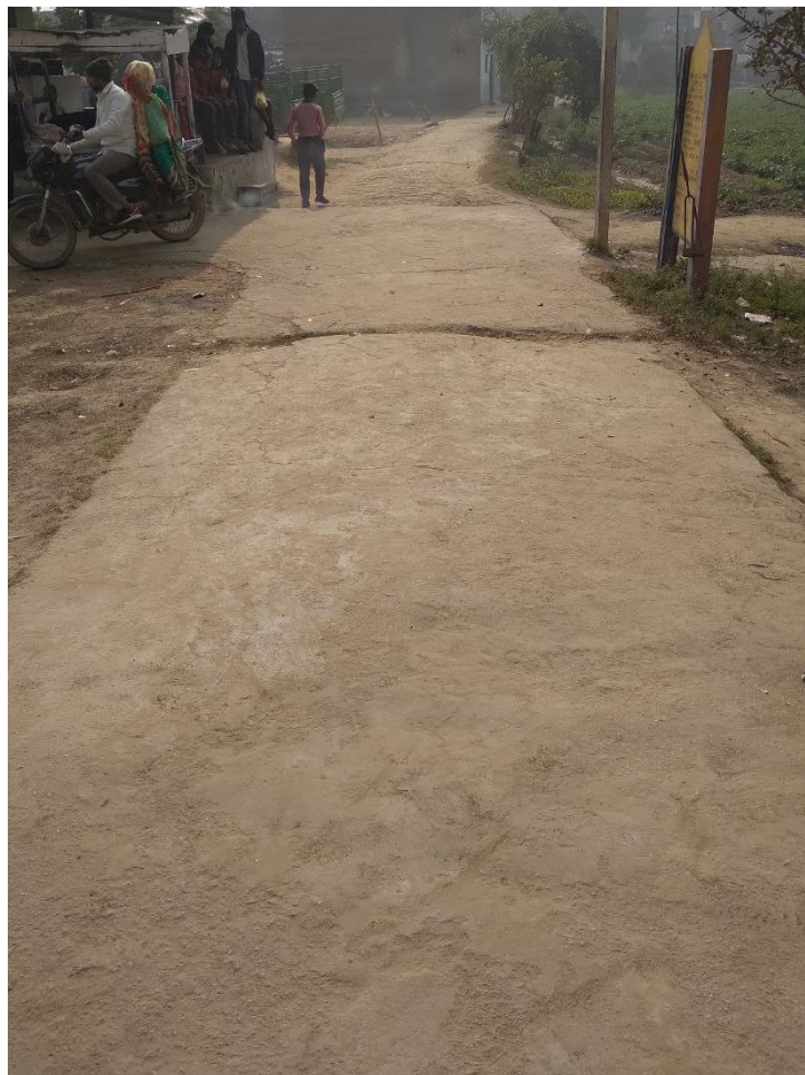
Fig. 3: Pucca Road that Connects Schools with main Road
