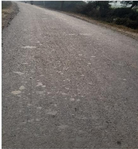
Fig 4: Main Road Connecting the Village to NH3
