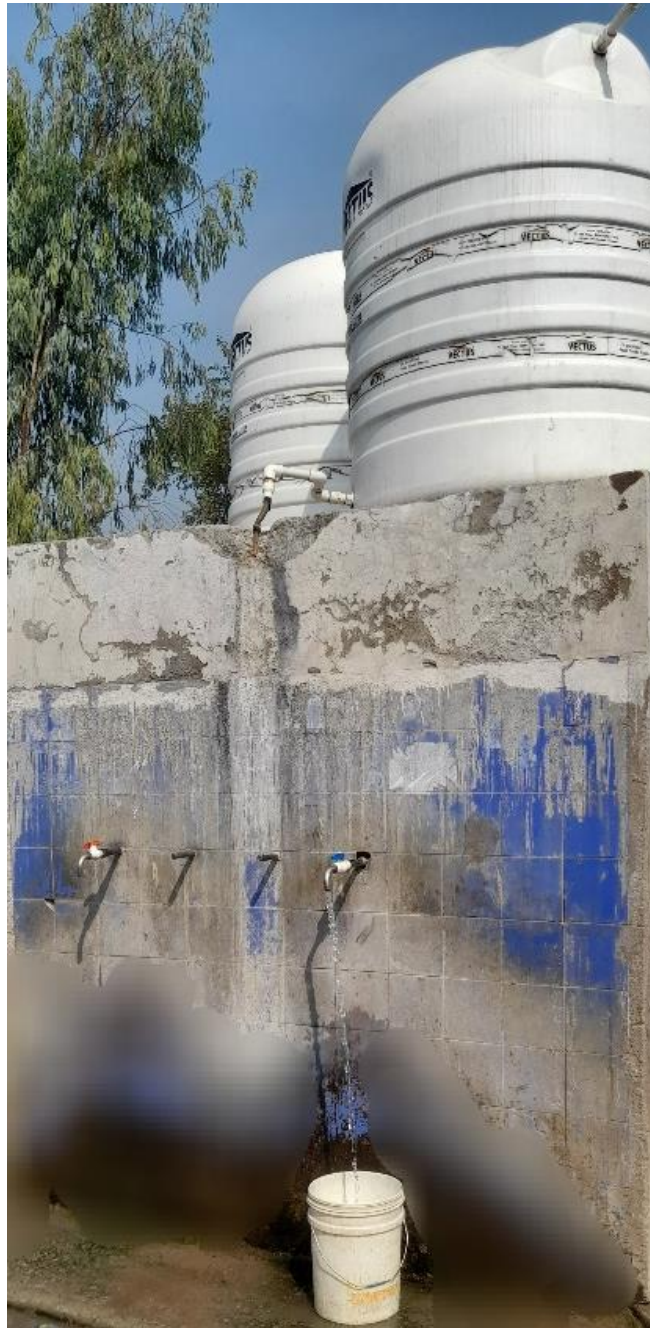
Fig. 6: Community tap water in the Village
