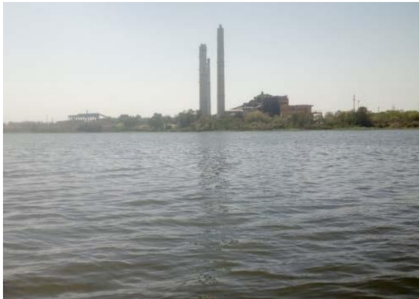
Fig 2: Stn.2 near the thermal power plant
