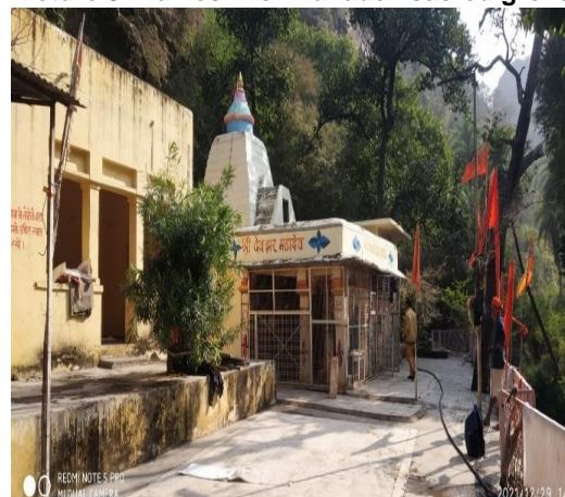
Picture 4: Shri Devjhar mahadev (Sathoor-Hindoli)
